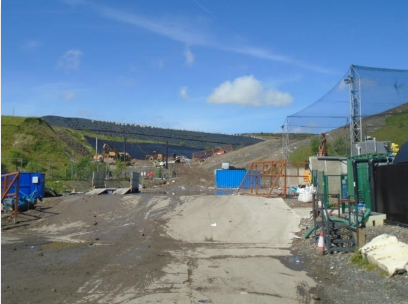
Site compound looking into landfill area
